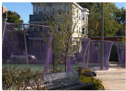
The project consists of a sculptural fence made of chain link fabricated in a serpentine sharp with sinuous curves. In this fence, the top and bottom rails are serpentine, and the pother posts are set purposely at angles to create a sense of rhythm and energy. The chain link fabric is stretched around the structure to create billowing curves.
